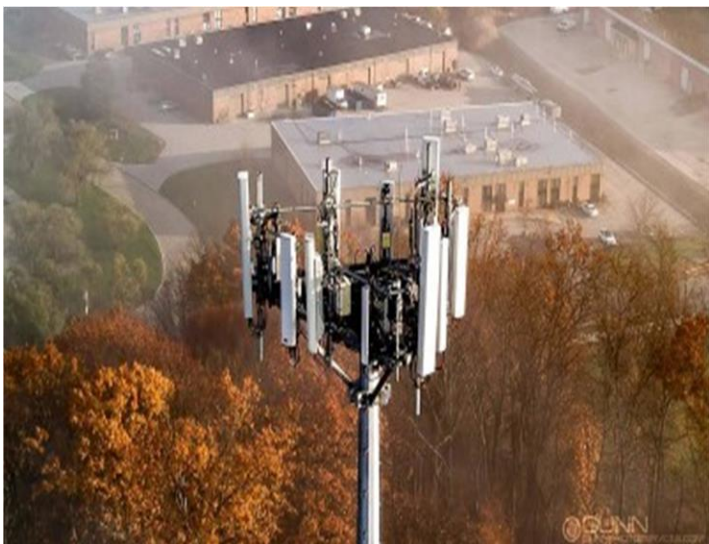
Vertical Structure Inspection
