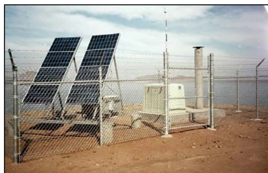
Figure 2. CGPS site at the East Dam
