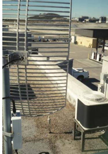
Figure 6. Remote CGPS site with antenna aimed toward backbone site (left) and backbone antenna on roof of building with LAN connection aimed at CGPS site (right).
