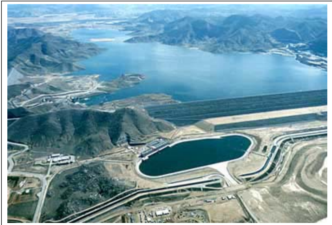
Figure 1. An aerial view from the west of Diamond Valley Lake in Riverside County. With a surface area of 4,500 acres and a storage capacity of 800,000 acre feet (260 billion gallons), the reservoir will provide six months of emergency supplies in the event of a major earthquake, provide additional water for drought protection and peak summer needs, and nearly double the region's surface water storage capacity ( Metropolitan Water District of Southern California , http://www.mwd.dst.ca.us/ ). Shown is the northern end of the West Dam and the smaller Saddle Dam. The West Dam is monitored in real-time by two Leica CRS1000 receivers, the Saddle Dam by one receiver. Altogether seven Leica CRS1000 receivers are deployed on three large earthen dams and at two reference sites located on stable rock close to the two larger (West and East) dams. (See Figure 2 for a map view of the GPS network).
